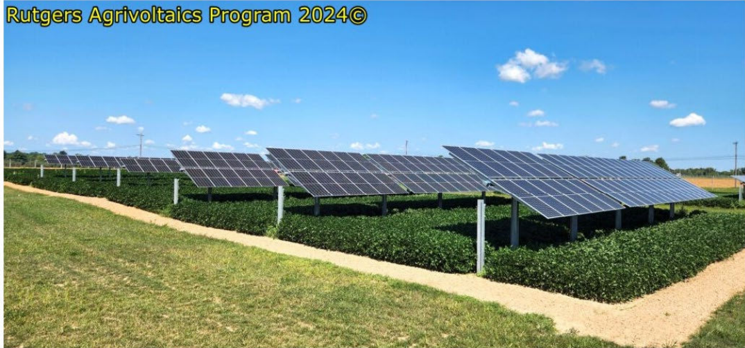
Figure 1. An image of the soybean trial near mid morning at RAREC in 2024. Note: the double AV panel block (closest) with the single AV block (in the background), followed by the control block (no panel) are facing east toward the sun.
