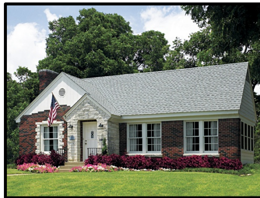
Cool Roof shingles don't look different, but a special coating cuts air conditioning costs.
