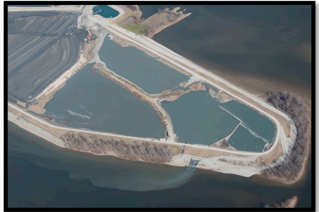
TVA's New Johnsonville coal ash pond, "Ash Island" releases untreated wastewater into the Tenn. River.
